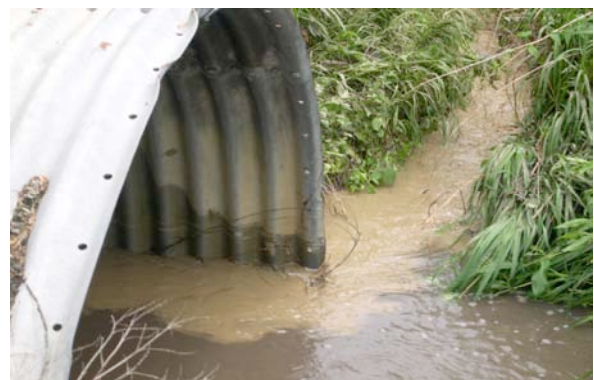
Above, sediment-laden runoff leaving a new housing subdivision, June 2007. Below, the same runoff flows quickly into a local creek.
