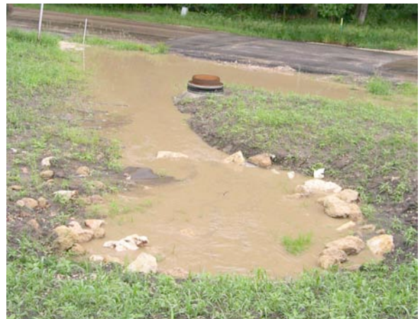
Above, sediment-laden runoff leaving a new housing subdivision, June 2007. Below, the same runoff flows quickly into a local creek.
